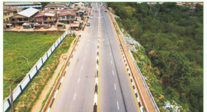
NEWLY COMMISSIONED PANSEKE - ADIGBE - OPAKO ROAD
