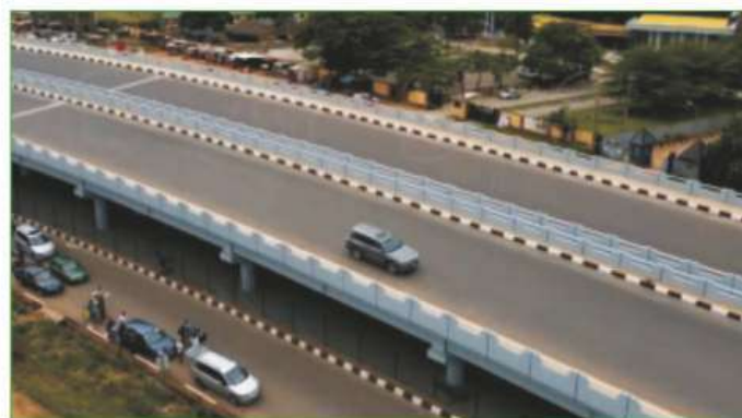
COMPLETED KUTO BRIDGE, ABEOKUTA
