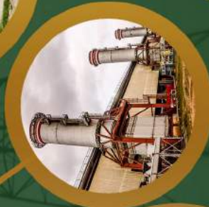
EGBEMA POWER PLANT Capacity: 360MW
